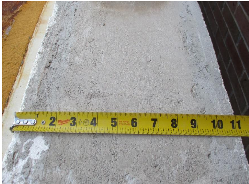
Photo No. 3 View of ICF Wall after Concrete was Placed
