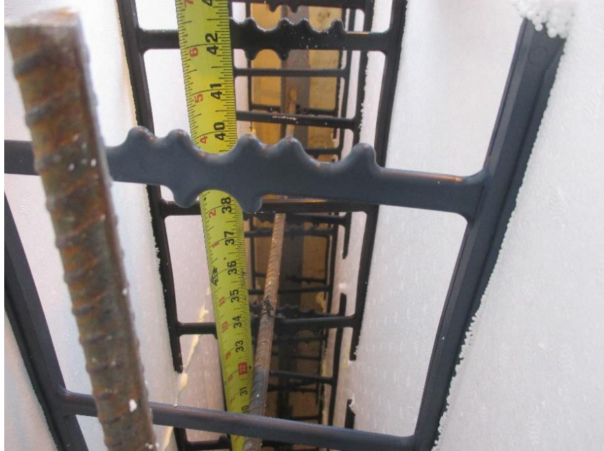
Photo No. 2 View of Inside ICF Wall before Concrete was Placed
