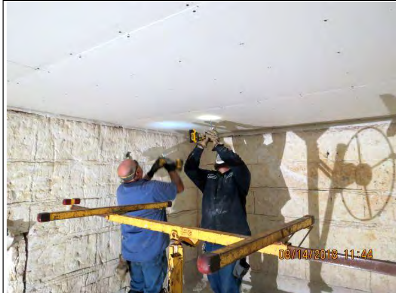
Photo No. 29 Installation of gypsum board
