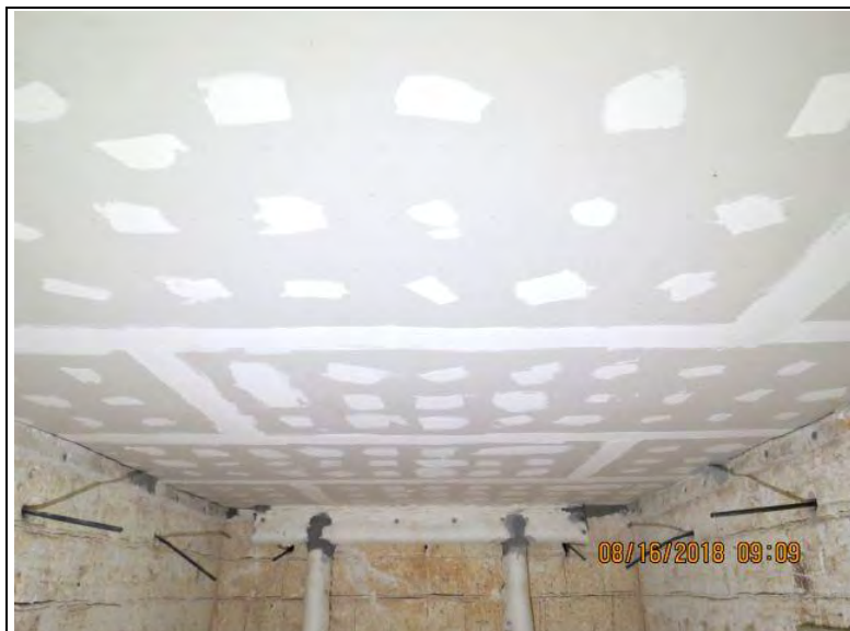
Photo No. 30 Exposed side – completed prior to fire test
