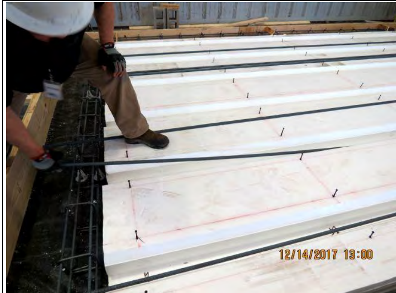
Photo No. 13 Installing tensioning member rebar
