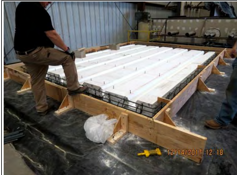
Photo No. 1 Construction
