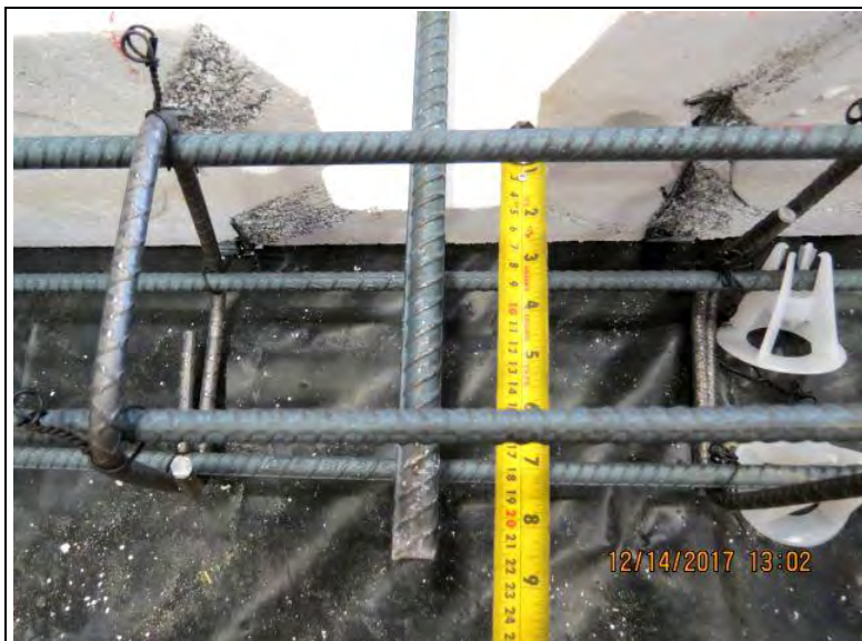
Photo No. 14 Installing tensioning member rebar
