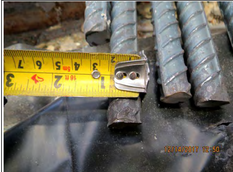
Photo No. 9 Tensioning member rebar
