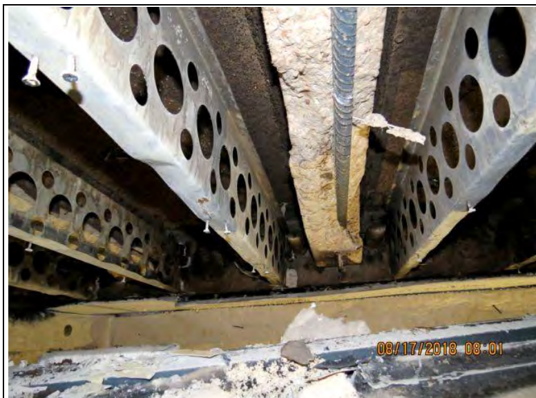
Photo No. 48 Post-test
