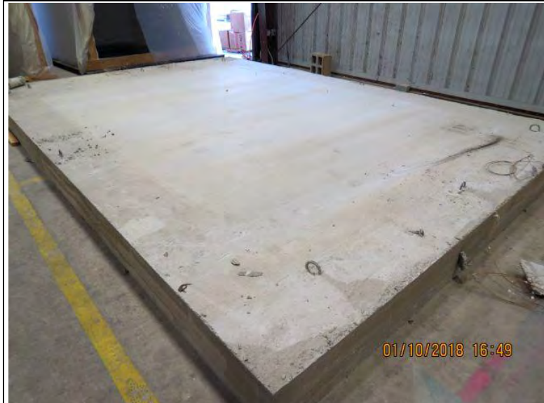
Photo No. 21 Completed assembly
