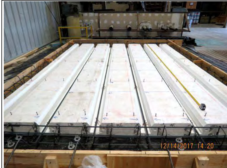
Photo No. 17 Tensioning member TC location layout
