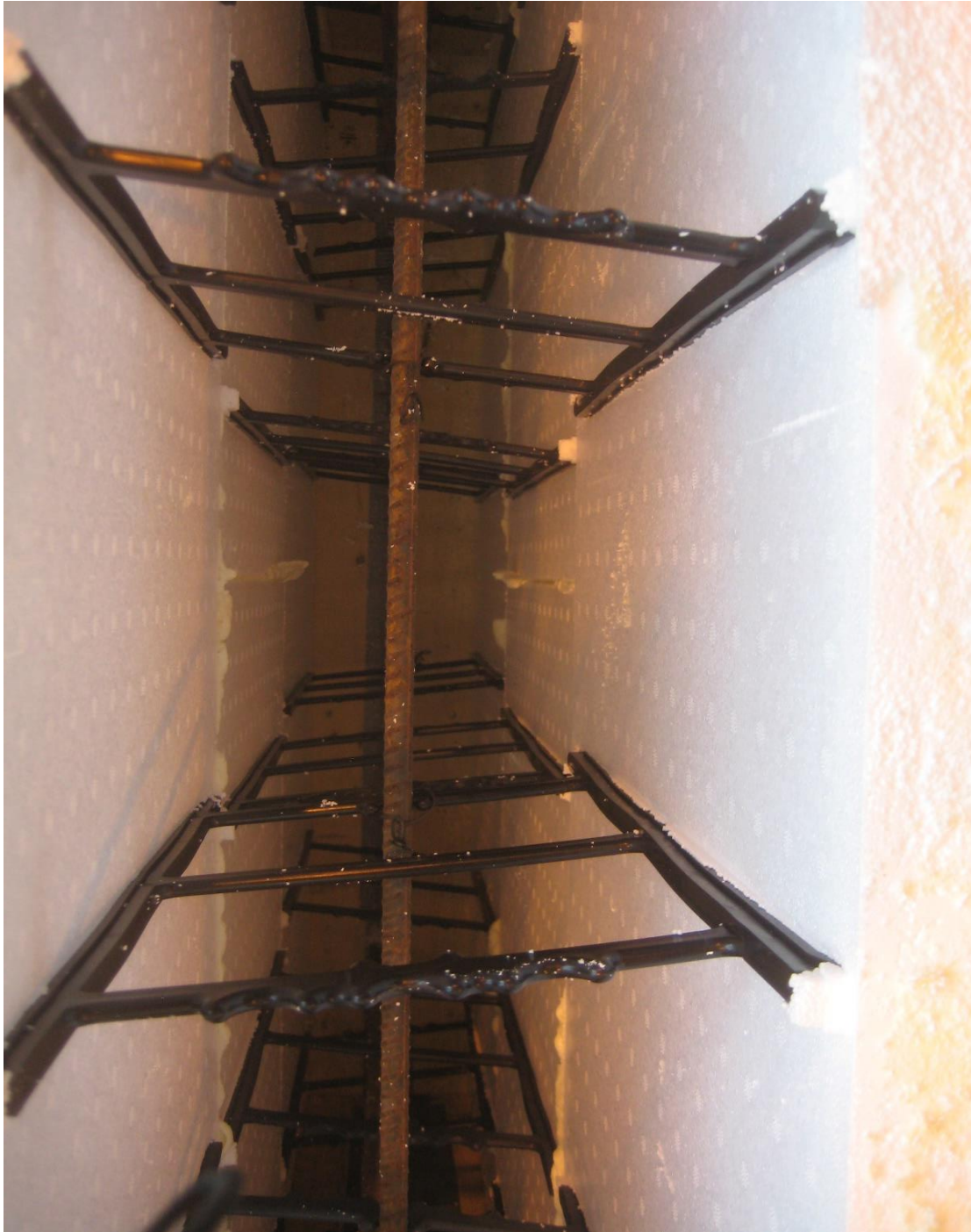
Photo #5, unit being constructed, before concrete pour
