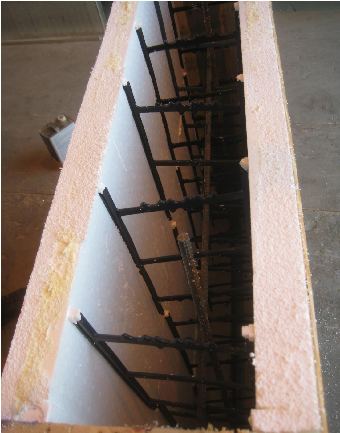
Photo #4, unit being constructed, before concrete pour
